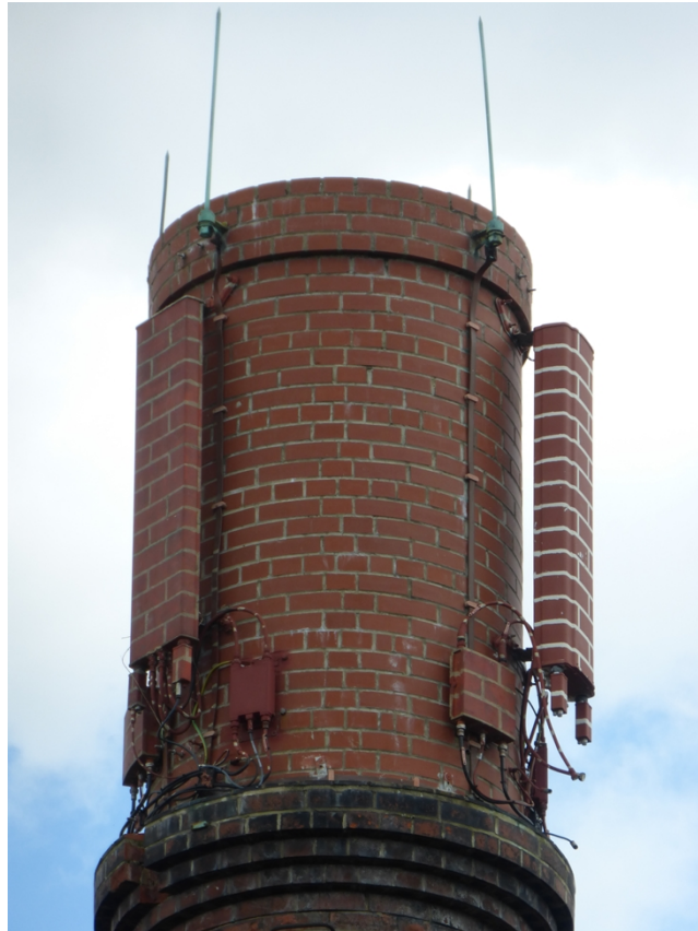
Example of existing antennas on the chimney.
