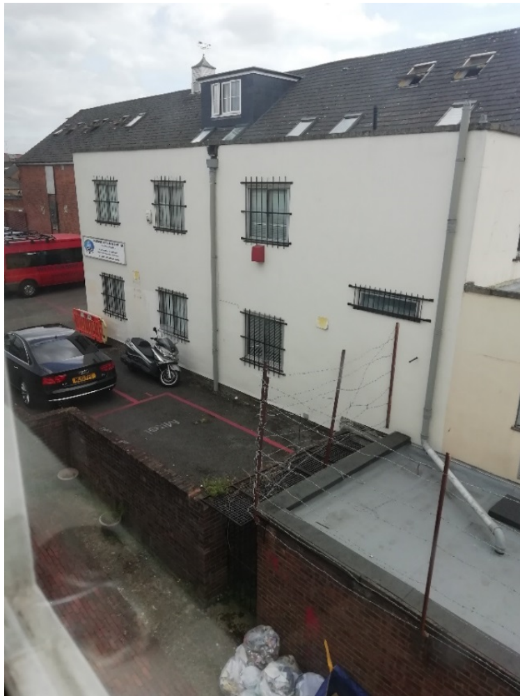
Figure 11 - View east from the second-floor window of RISC offices along Sims Walk
