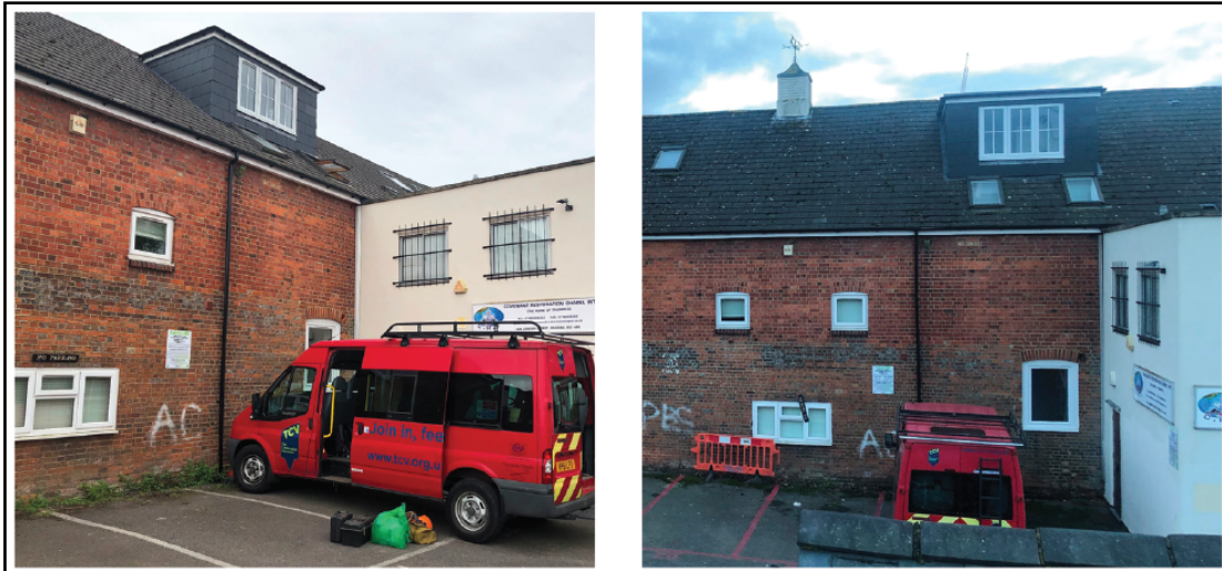
Figure 6 - Existing windows at rear of London Court facing car park
