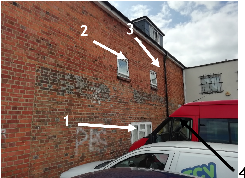
Figure 13 - Existing windows to the rear elevation of London Court
