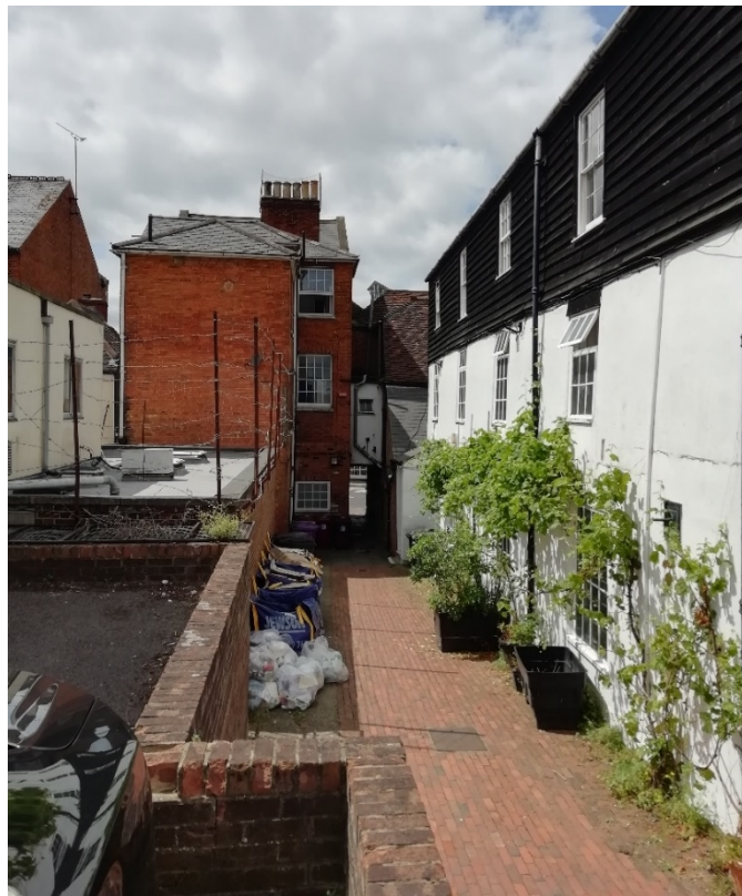
Figure 9 - View west along Sims Court (RISC offices to the right)
