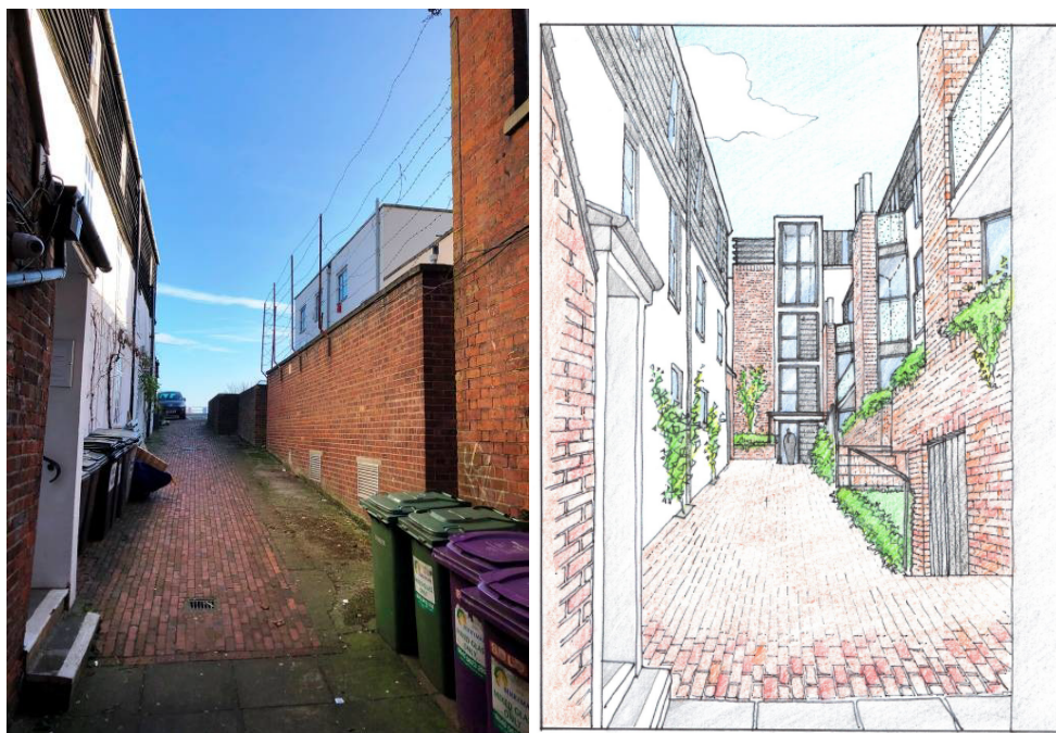
Figure 6 - View up Sims Court eastwards (existing photo and proposed sketch) taken from Design and Access Statement
