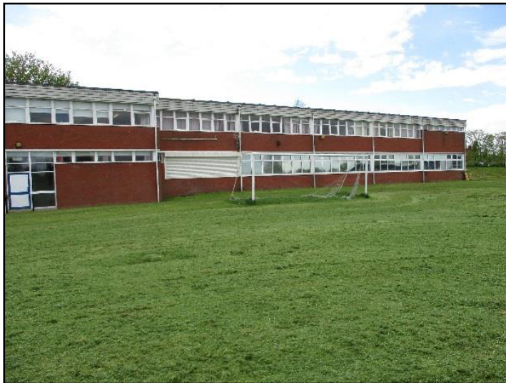
Figure 6 - View across pitches towards existing building
